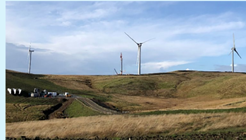
Tralorg Wind Farm
